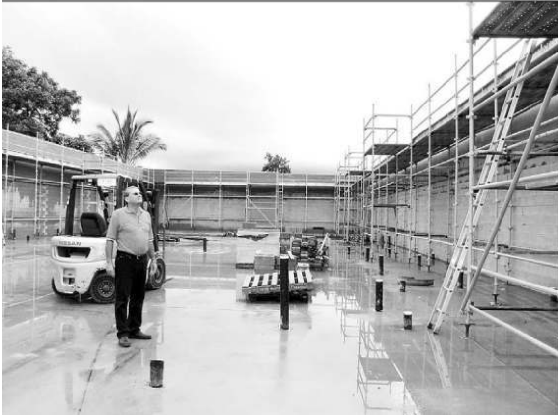
Owner Tony Zaghini inspects work on the new supermarket yesterday
