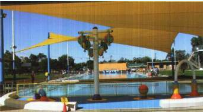
Cobar Memorial Swimming Pool after RenovAction® upgrade
