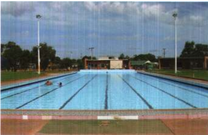
Cobar Memorial Swimming Pool before RenovAction® upgrade
